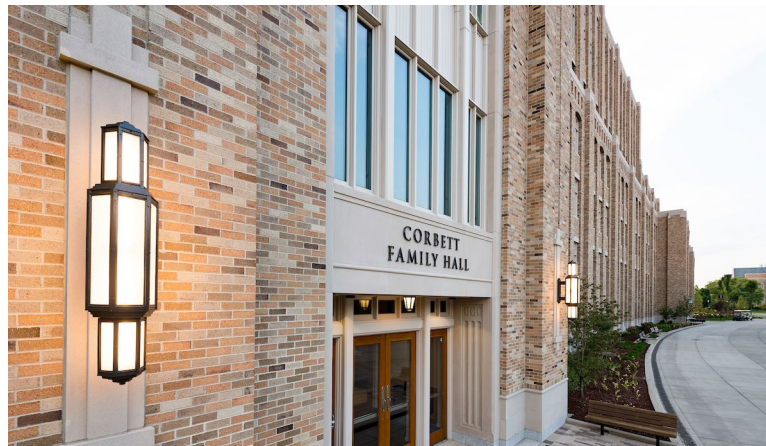
Corbett Family Hall - Notre Dame Southside Precast Products
