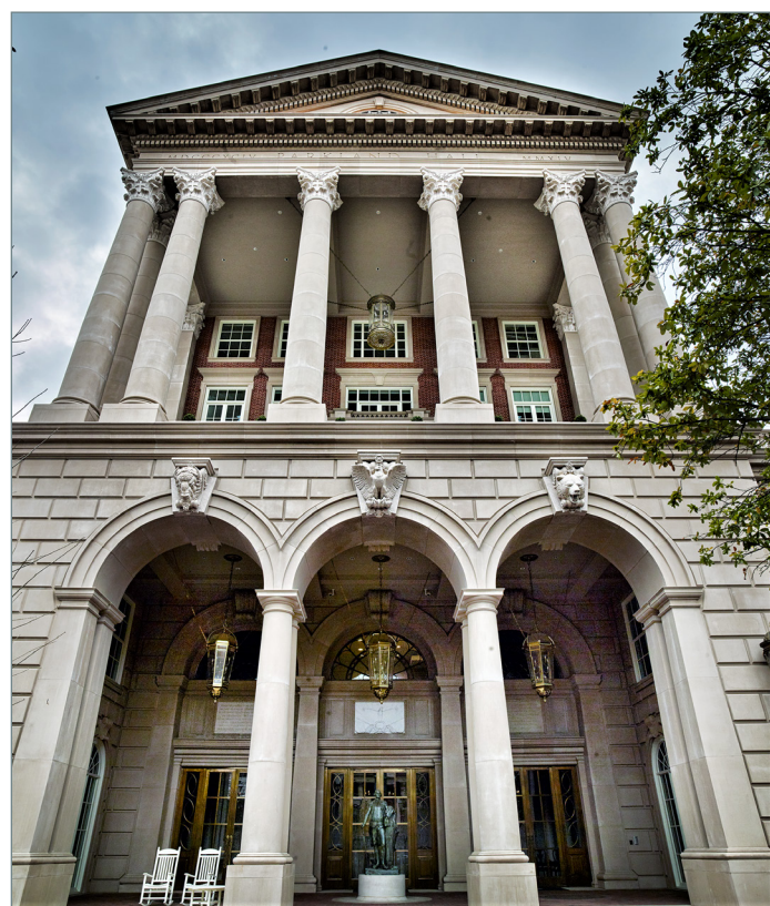
AAS is quite proud of the enormous Corinthian capitals it crafted to sit atop 16-foot-tall columns at the Old Parkland West campus in Dallas. The company was aided by a 3D Revit model and CNC-generated molds to make the columns to scale. Photos courtesy of Advanced Architectural Stone
