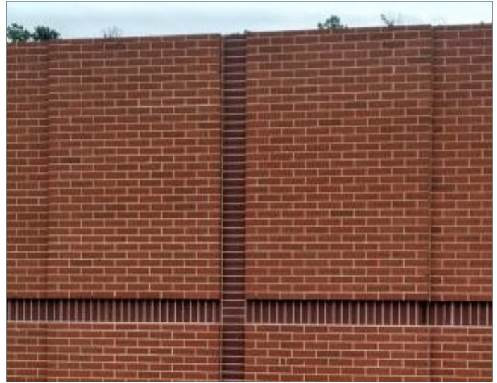
With the right form liner, brick patterns may vary throughout the panel while still emulating a consistent look. Seen here, recessed and protruding sections combine for an appealing look. Photo courtesy of American Stone Virginia
