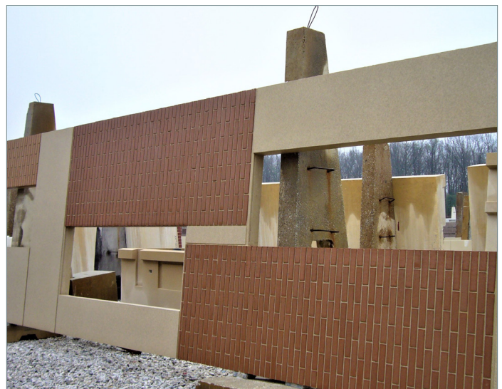
In some buildings, a stacked and spandrel-column system enables precast panels to support the panels above them. Photo courtesy of American Stone Virginia
