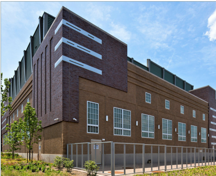
Thin brick is a popular choice for architectural projects. The Pepco building in Washington, D.C., features thin brick-clad panels made by Arban & Carosi with brick manufactured by Endicott. Photo courtesy of Endicott
