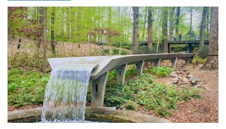
not only vertically but horizontally as it dropped in the terrain. In addition to matching radian, there is a fall of approximately 1/4" - 3/8" in each joint.
