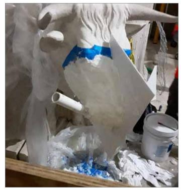
Step 4 – After removing the hard shell and rubber mold, drill a series of bolt holes to tightly secure the mold system to the areas of repair. Pour the repair material into the pour hole. Tap the hard shell to consoladate the repair material and remove any air holes. After 12-24 hours remove the mold system and perform any minor touch-up to the repair area.
