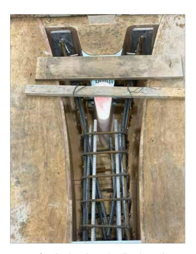
amount of steel in the columns that allow the product to take tremendous loads. The maximum flume section was roughly 16 feet and cantilevered five feet straight section into the pond. They mounted a stainless-steel diffusion plate that was grounded in the front column.
